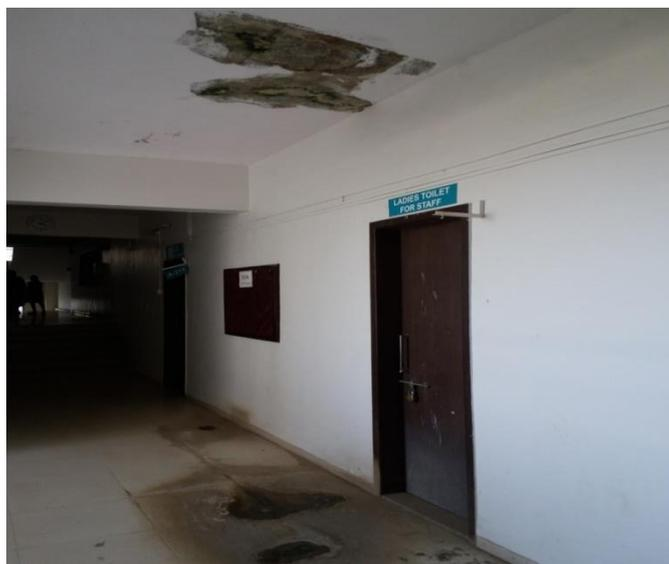
*Figure 1. Location of the leakage*
